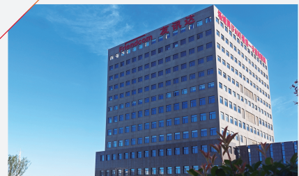
△ Wuhan Industrial Park
